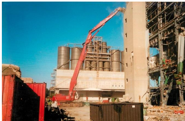
Demolition site. Source: VERAS
