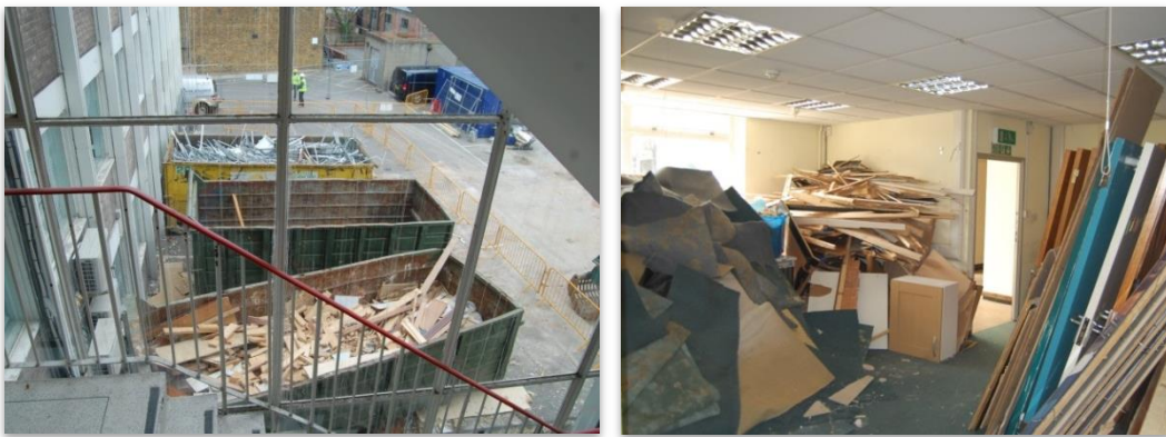
Source separation at a demolition site, Source: UEPG
